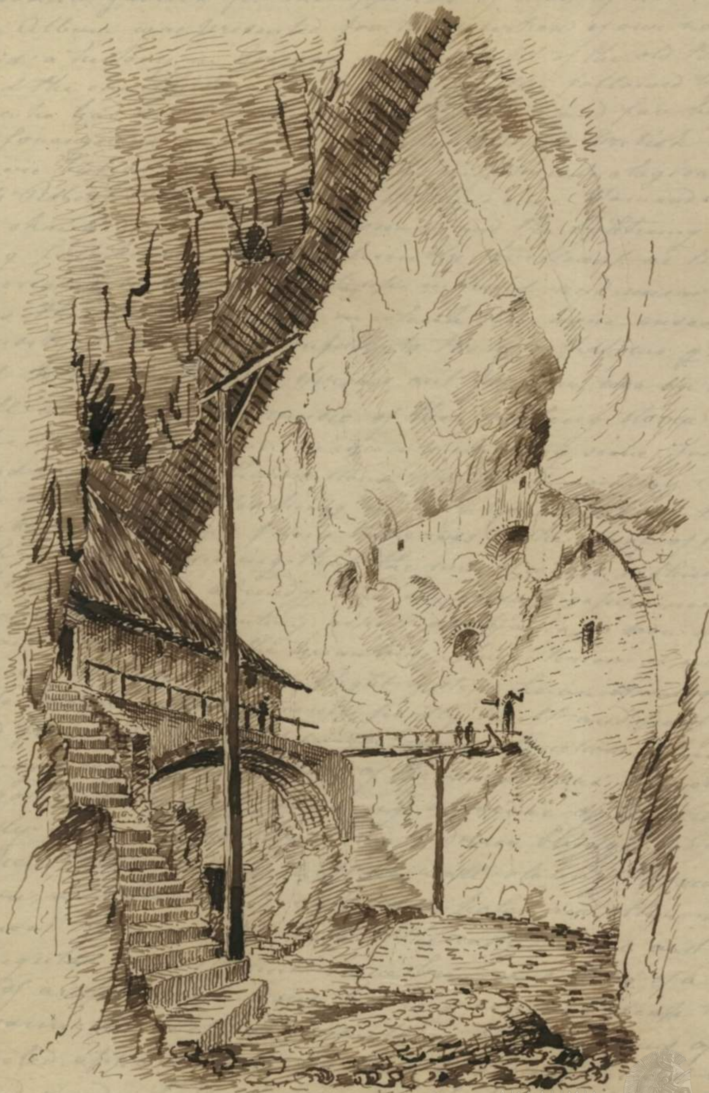
Entrance to the fortified cavern Luigi.
